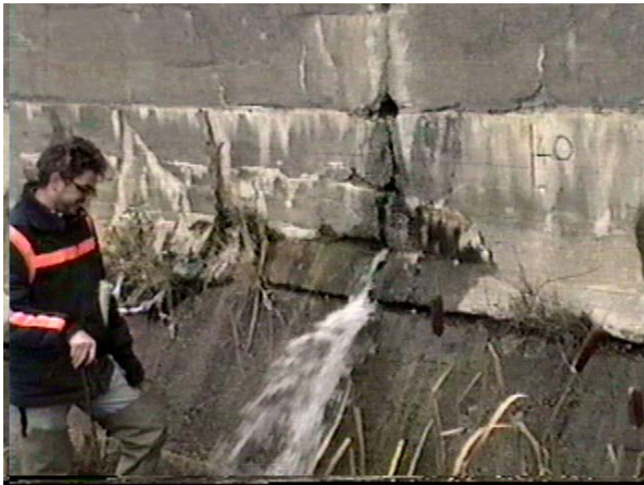
Fuites Seepage (Leaks)
