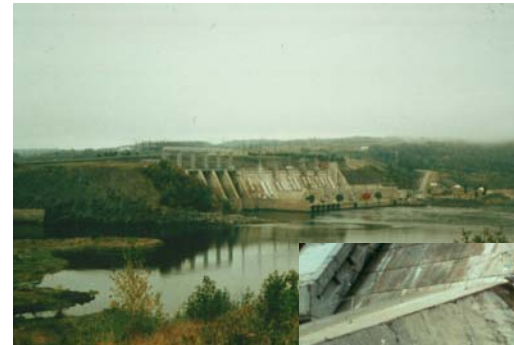
Slot Cutting at Mactaquac G.S. New Brunswick
